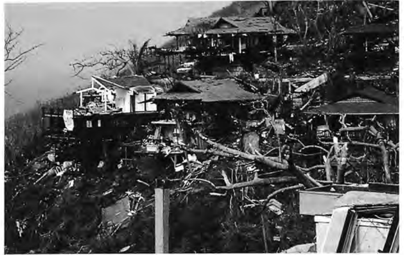
Figure 3.30: Wind speed-up in St. Thomas during Hurricane Marilyn produced extensive damage to residential and commercial structures.
