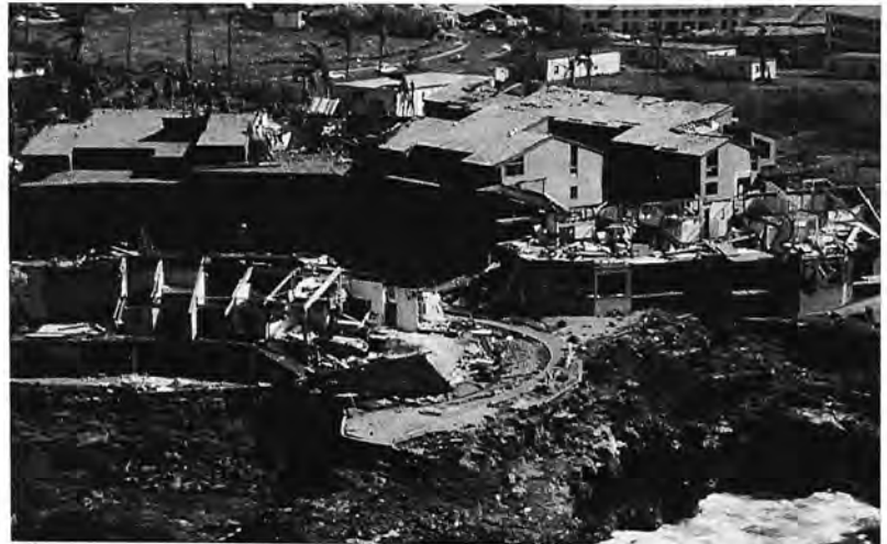
Figure 3.31: Localized damage due to wind speed-up Poipu Beach, Kauai due to Hurricane Iwa (1982).
