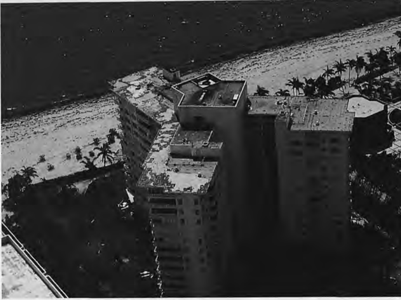
Figure 5.30: This Y-shaped hotel suffered extensive damage during Hurricane Andrew.
