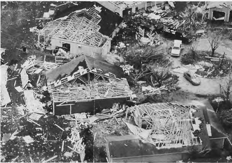
Figure 1.5: Aerial view of damage at Country Walk, South Miami, FL, due to Hurricane Andrew. Note dominoing of roof trusses after sheathing is lost.
