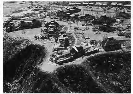
Figure 3.35: Localized damage due to wind speed-up; Princeville, Kauai, Hurricane Iniki, 1992.
