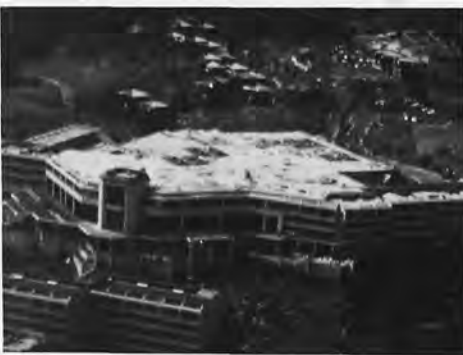
Figure 6.4: This hotel was out of service for four years after hurricane damage to the roof.
